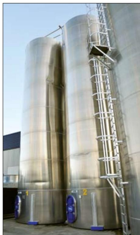
*PET storage vessels showing wall buckling caused by silo quaking.*
