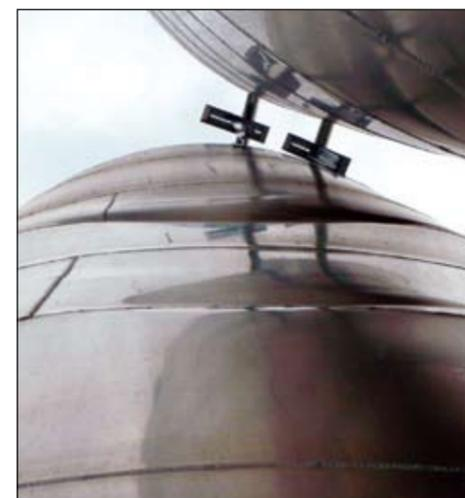
*Vertical view showing the distortion from cylindrical shape caused by silo quaking.*
