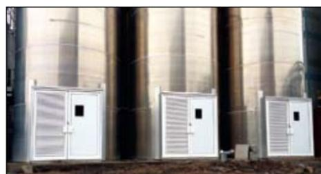
*These Barton silos (left) have been treated with a special coating so as achieve reduced visual impact in an area of natural beauty; they are fitted with double doors (as shown above on a different Barton silo installation) to allow access to the base area.*
